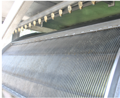
Drum is cleaned by water or recycled effluent
