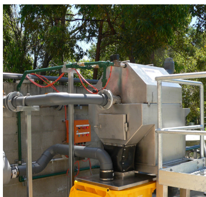
Mini-Milliscreen™ installed at a winery.
