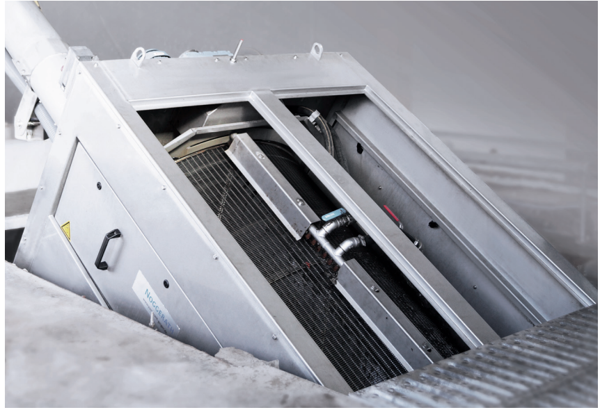
Rotary Drum Screen installed in channel
